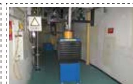
Temporary Shielding Device for Radiation Hotspot
